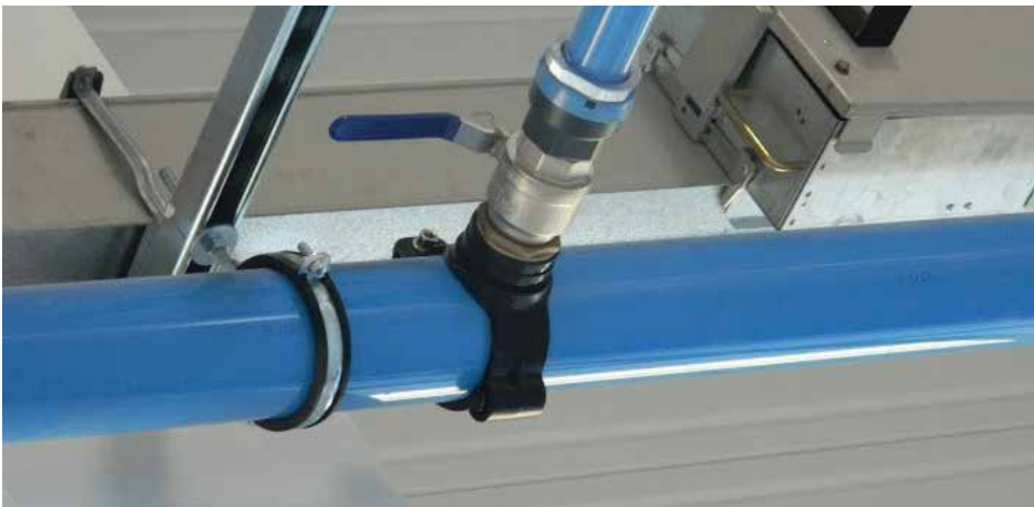
Typical Application for Saddle Branch
