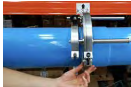
Step 6: Release UnipipeEZ Install Tool from pipe.
