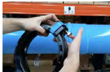
Step 7: Loosen bolts on coupling to put around the pipe on the groove.
