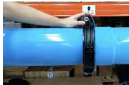
Step 8: Tighten bolts on coupling once the coupling is placed on UnipipeEZ.
