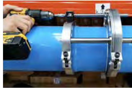
Step 5: Use power drill to close the UnipipeEZ Install Tool and insert pipe together.
